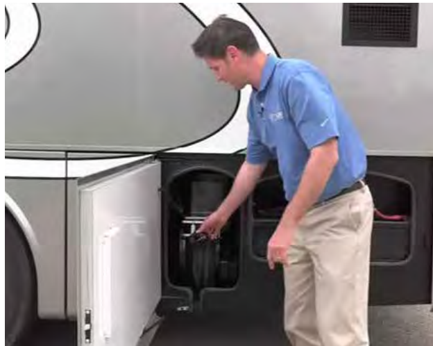
50 amp shore power cord attached to an electrical-powered reel.
