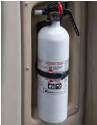
Typical Class B-C fire extinguisher
