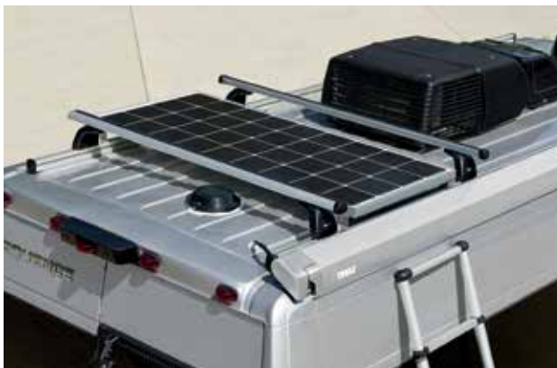
Typical solar panel installation
