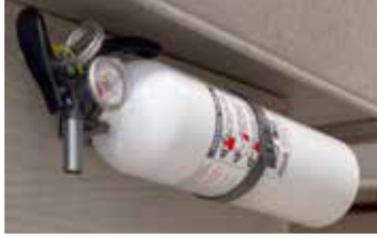
Typical Class B-C fire extinguisher
