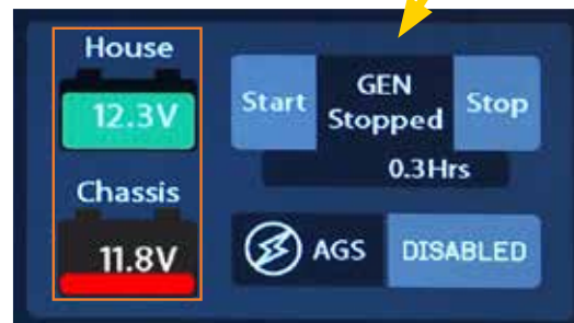
Typical multiplex main control panel. Basic electrical system monitoring is usually located on the main menu (Home) screen.
