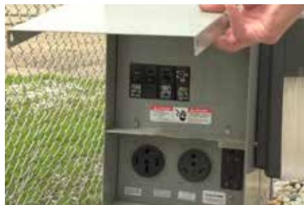
4-prong 50-amp shore power cord (left) and 3-prong 30-amp shore power cord (right)
