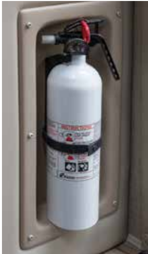
Typical Class B-C fire extinguisher
